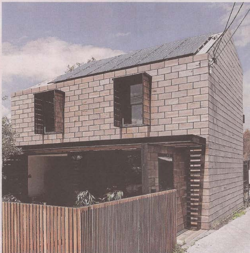
Clever effect: The facade features silver top ash tiles, laid like stonework on steel framing. Photo: Andrew Wuttke
